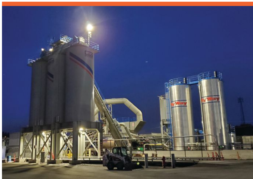
A year-and-a-half of planning was put into All Roads Construction’s purchase, assembly and commissioning of its new Gencor 300TPH Skidded Asphalt Ultraplant.
