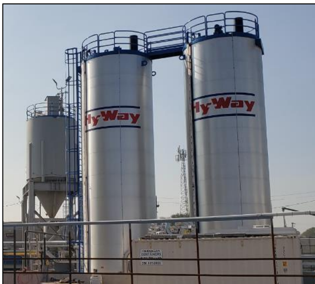
Figure 3: Asphalt cement (AC) storage tanks
